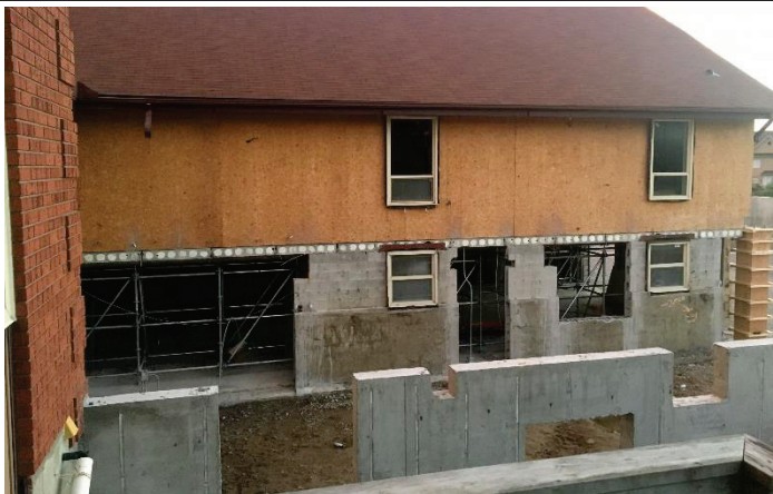
Openings cut in original foundation to connect to new section
